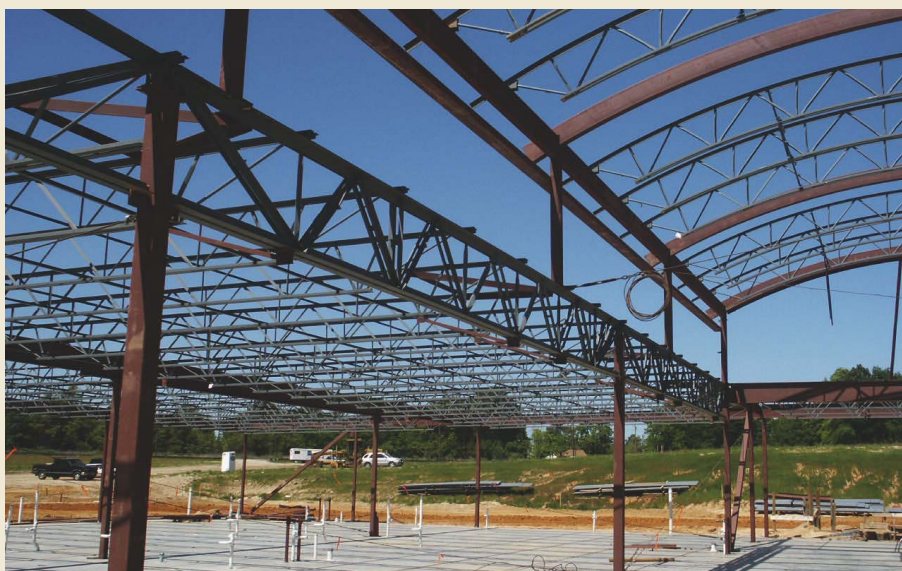
Open web steel joists can be adapted to a variety of geometric configurations.
