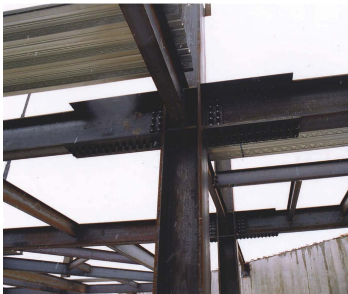
A completed bolted moment girder connection with top and bottom flange plates at Heart Hospital.
