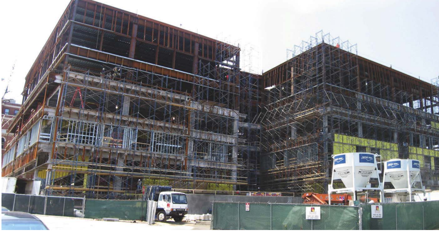
Maine Medical Center's Women and Infants Building in Portland, Maine (scheduled for completion in 2008) is a five-story welded steel moment frame with capacity for two more stories.
