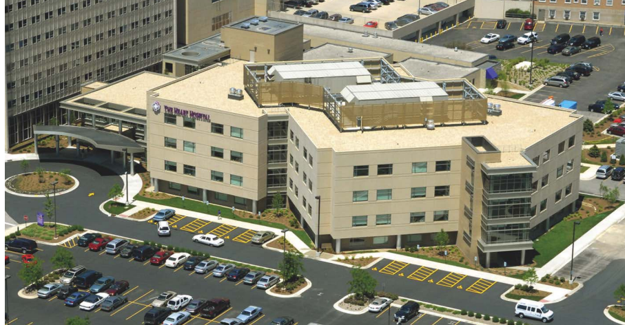
SwedishAmerican Health System's Heart Hospital in Rockford, Ill. is a four-story bolted steel moment frame with capacity for two additional stories.
