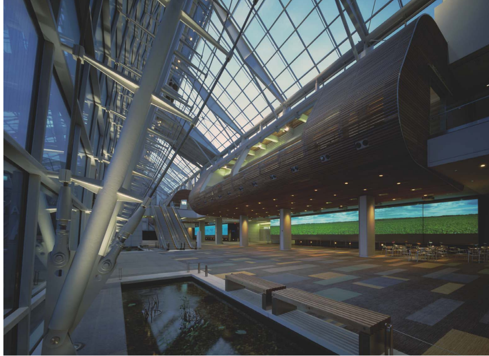
Vertical "fishbone" trusses (at left in photo)—consisting of round HSS, cruciform cross-section arms, and tension cables—support the glass enclosure of the pre-function space.
