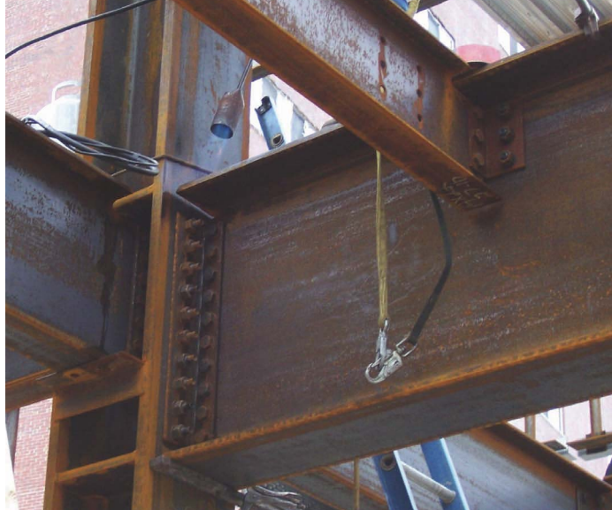
Preheating top flange of moment girder before welding in cold weather conditions at Maine Medical Center.
